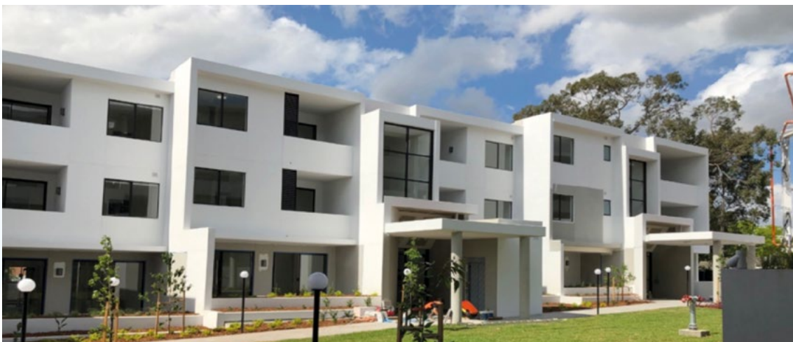
The Women's Housing Company and the Department of Communities and Justice worked closely to deliver new social housing for older women in Pendle Hill
